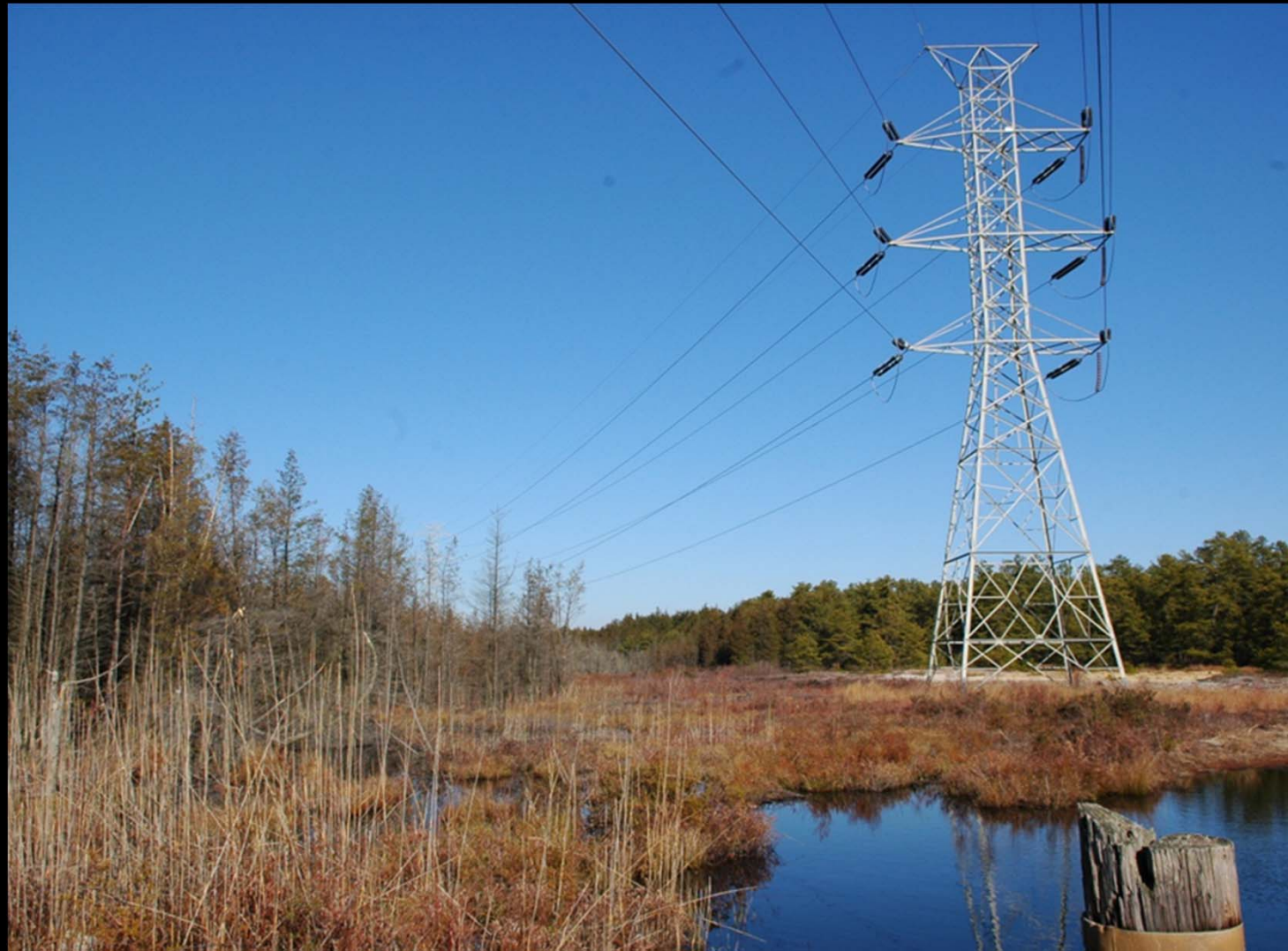
Wetlands spans on a JCP&L line in Berkeley Township
